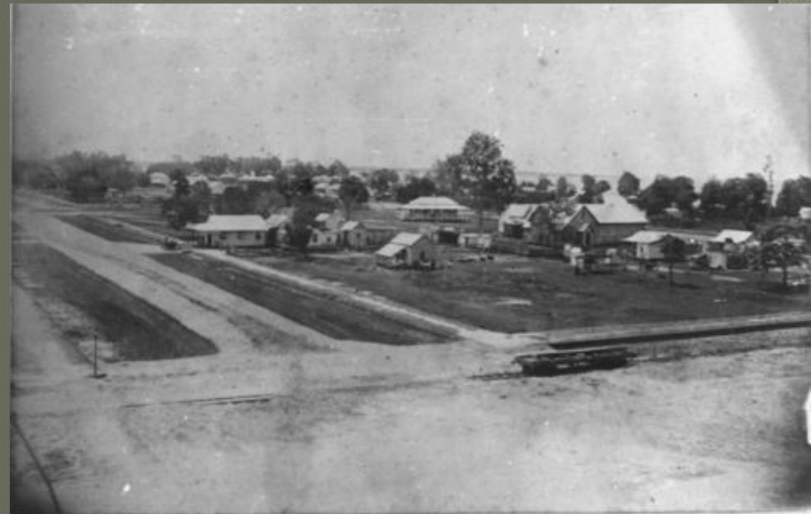
Sheldon - Lake St. Looking North
