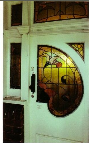
Above left A late Federation doorway, evidenced by the tapering architraves and the high-waisted door. Note the use of the double-reeled and ovolo profile to the architrave head, top of the skirting, door moulds and the lower architrave cut-out.
