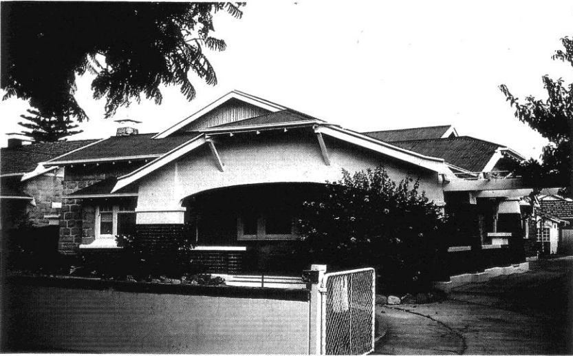
◁ 532 House, Ormond Grove, Toorak Gardens, SA. Architect and date unknown. A stone version, with brick-and-render verandas, and typical sharp roof edges.
