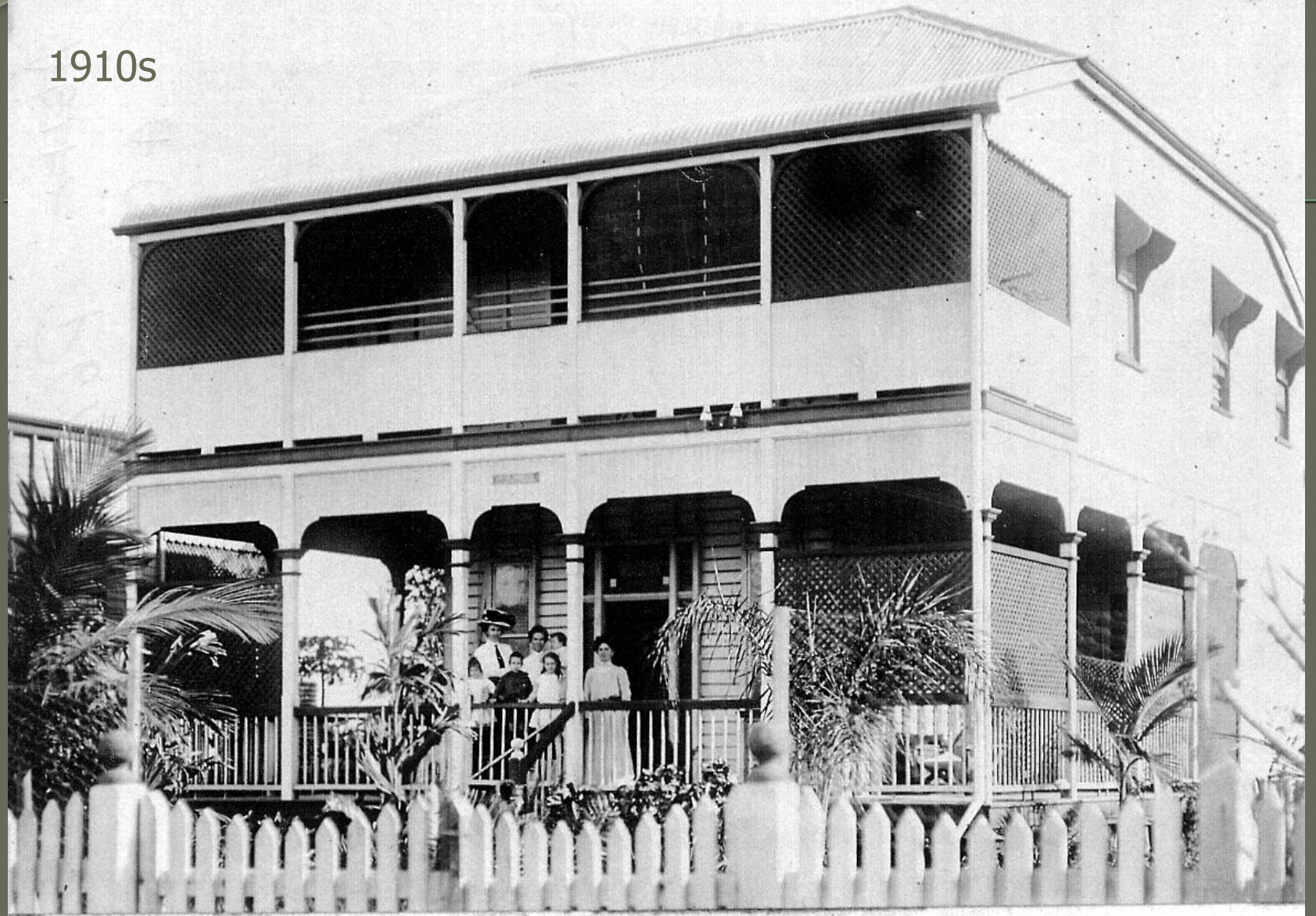
Weatherboard or chamferboard (external) walls Straight window shades (earlier – curved or bullnose) Hipped roof rather than pyramidal
