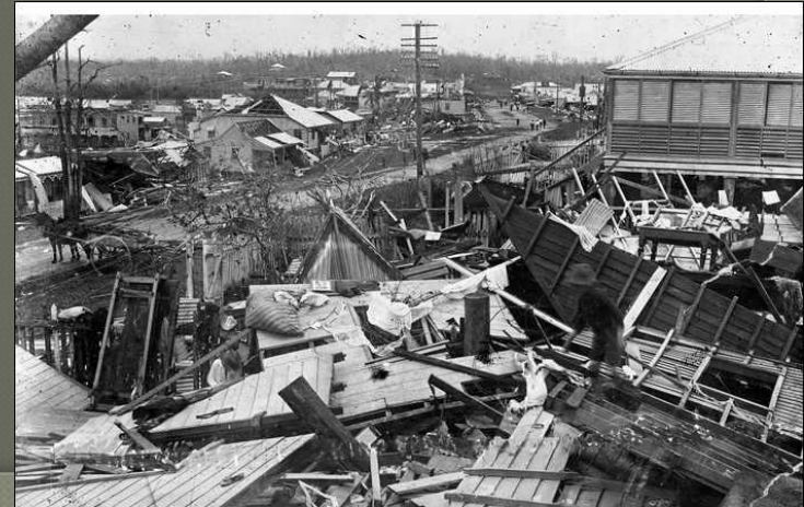
Destroyed house, 1918 cyclone, Innisfail
